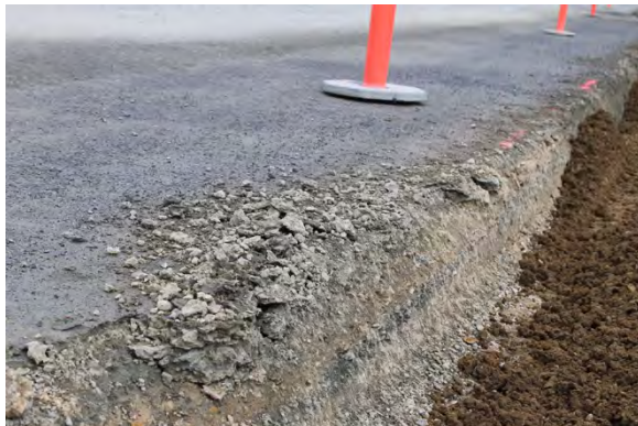
Figure 3.1 - Section boxed out to 250mm
