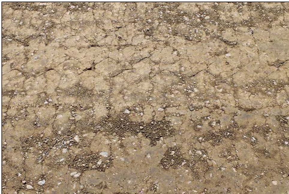
Figure 5.4 - Over compaction surface cracking
