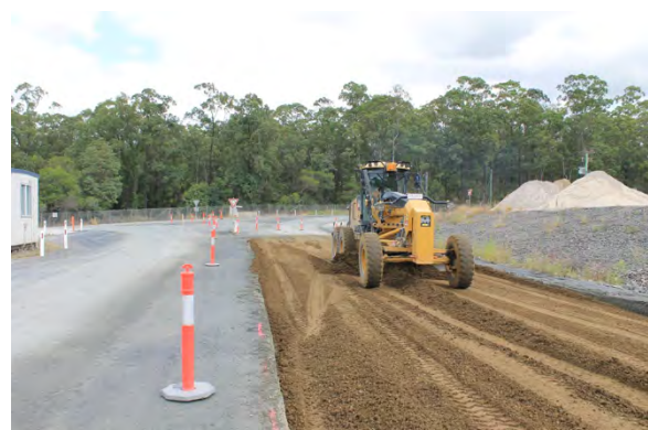
Figure 3.6 - Material placed and spread
