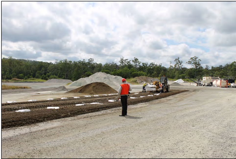
Figure 5.2 - Application of Solidry 25kg bags
