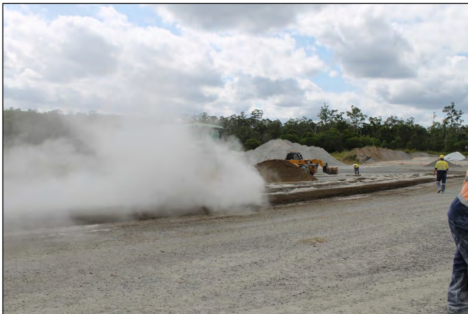
Figure 5.3 - Solidry dusting from harrowing
