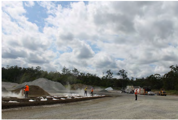
Figure 3.7 - Material treated with Solidry
