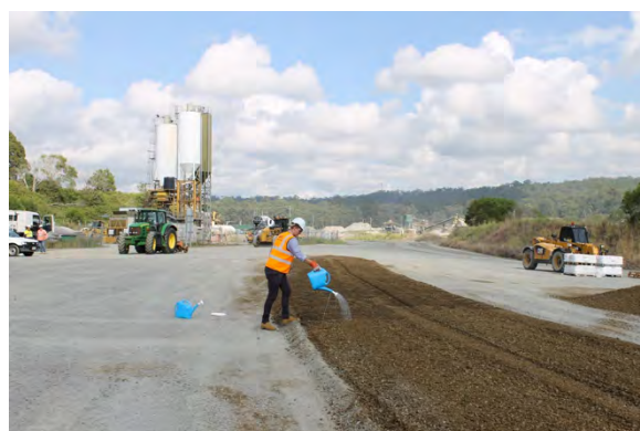
Figure 3.3 - Material treated with C444
